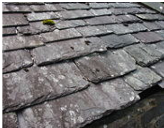
A Slate Roof
